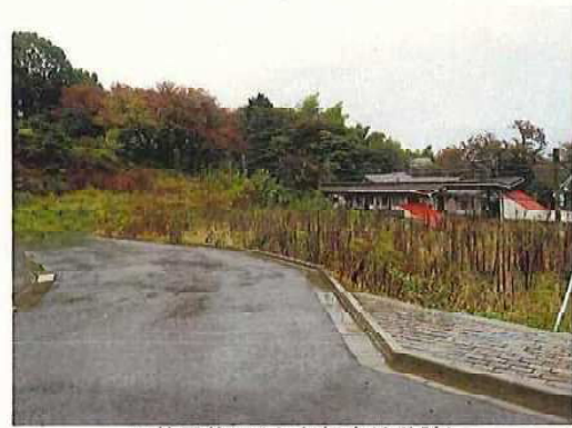
18放置状況(上多賀宅地分譲) 2009/11/11 11:27:05
