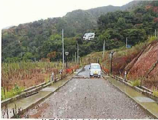
19放置状況(上多賀宅地分譲) 2009/11/11 11:31:05
