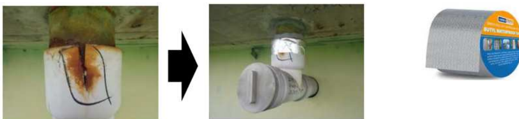
図-7.4 点検時の簡易補修の例②
