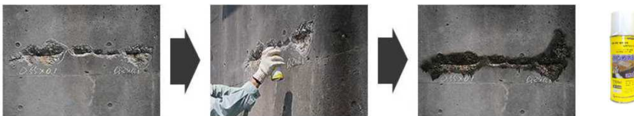
図-7.3 点検時の簡易補修の例①
