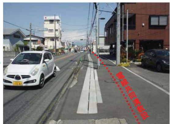
[電線共同溝敷設完了（抜柱前）]
