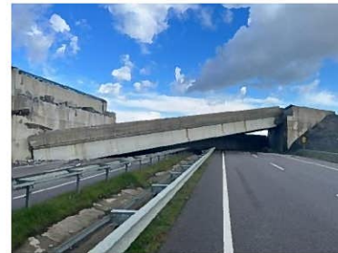
Overpass Bridge collapsed due to permanent ground movements
