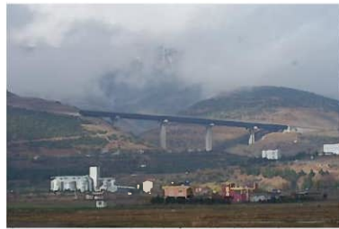
Turgut Özal Viaduct
