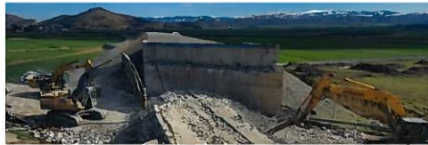
Overpass Bridge collapsed due to permanent ground movements
