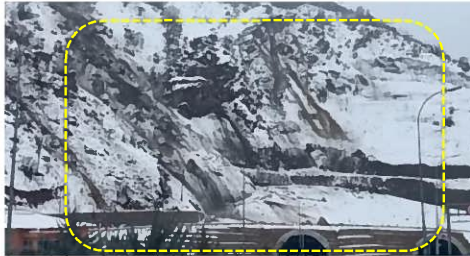
Traces and Rockfalls above the portals of new Erkenek tunnels
