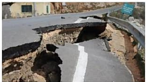
Longitudinal Separation cracks between clay core and rock/earth fill
