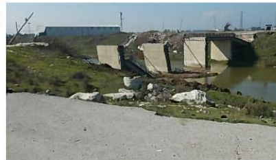
Bridge collapse due to pier settlement due to ground failure (Antakya)
