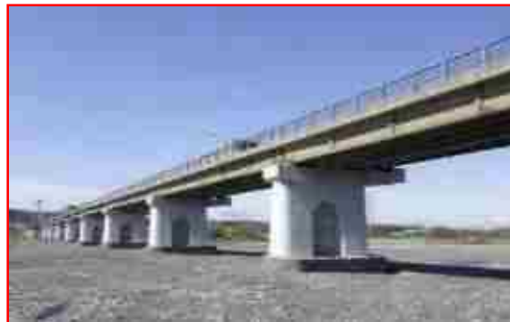
橋梁の耐震補強
