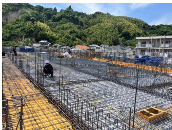
B棟4階床配筋
