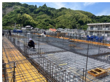
B棟4階床配筋
